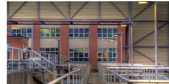
Water Recycle System Control Room
